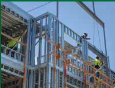
STEEL FRAMING @ KA MALANAI, KAILUA
